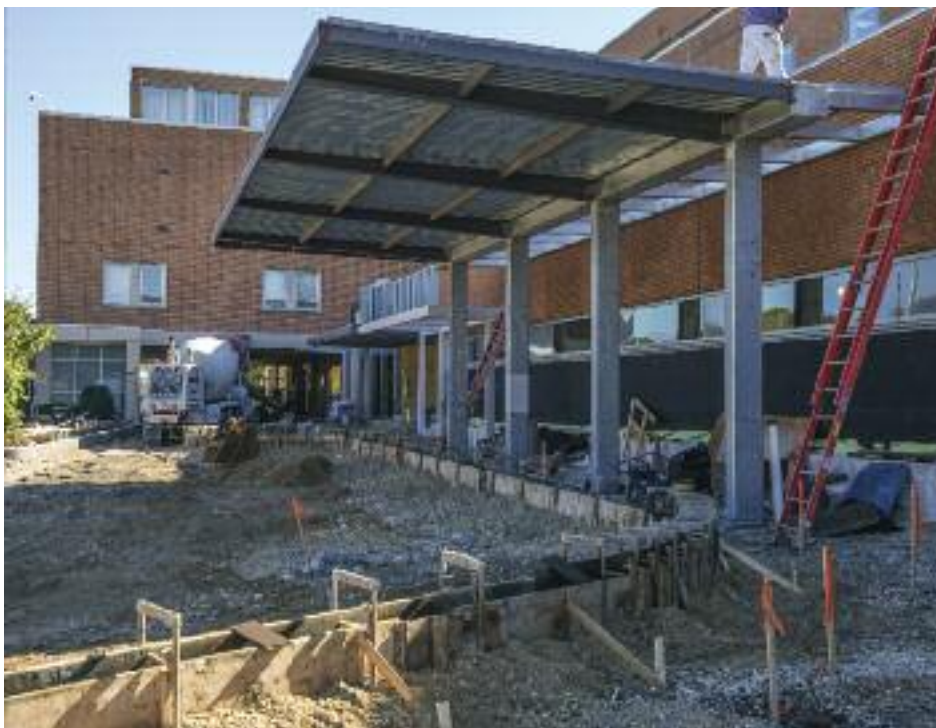
Exterior of new ED transforms daily while care continues inside.
